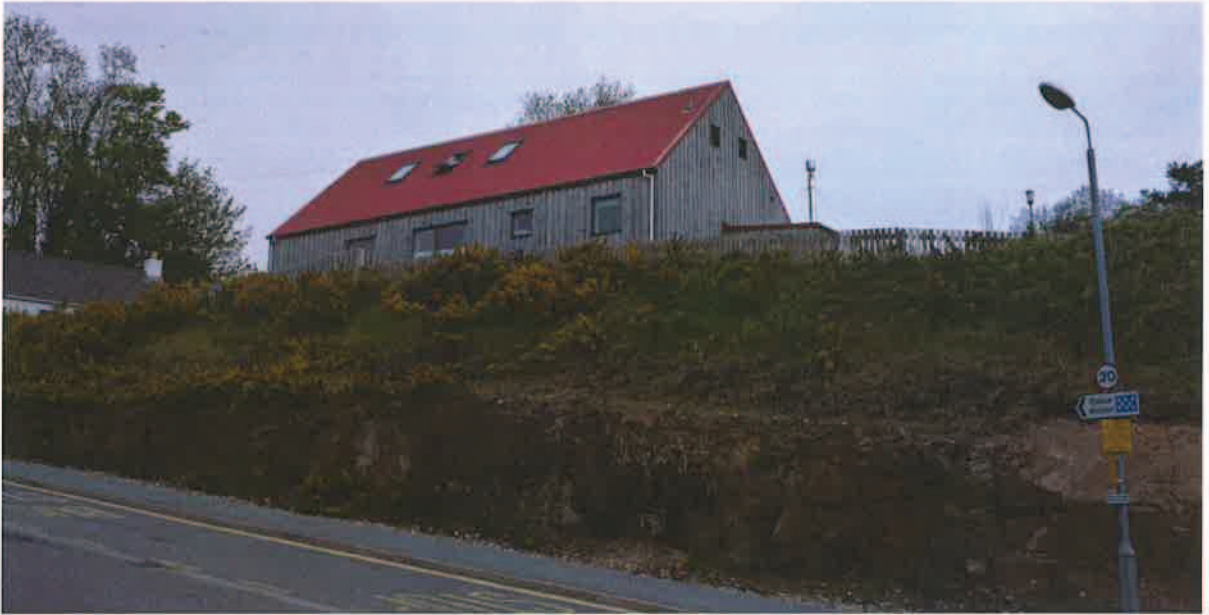
Figure 8 : New Primary School Building on periphery of Conservation Area
