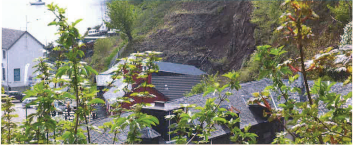
Figure 1 : Macgochans Pub, Tobermory - Original fishermans cottage extended (significantly) with a large profiled sheet roof and timber cladding to the rear of the building
