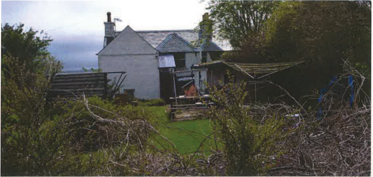
Figure 18 : Various materials used (breadalbane St)
