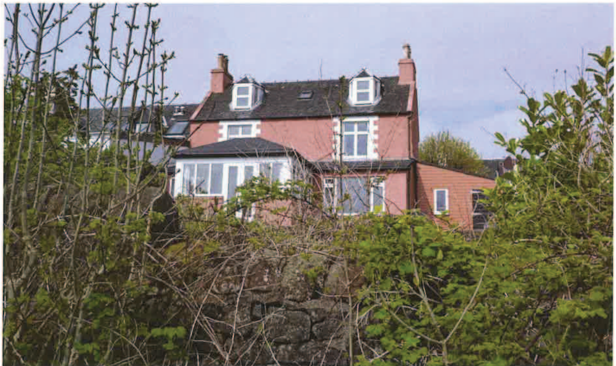
Figure 27 : Timber Sunroom (felt roof) and Timber side extension (Breadalbane St)
