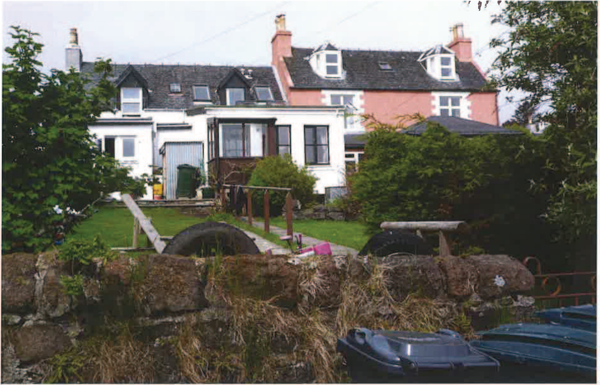
Figure 26 : Timber Porch, felt roofs (Breadalbane St)
