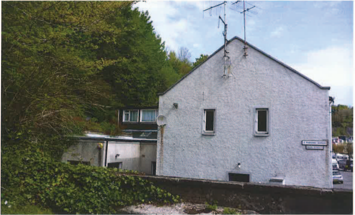
Figure 5 : Timber Clad, Profiled metal roofed extension to rear of building on Main Street, visible from main road
