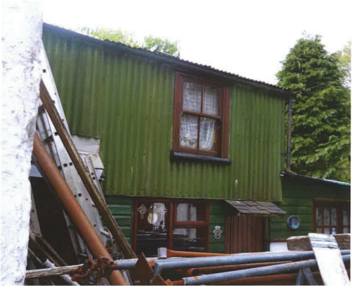
Figure 20 : The old Jail house - Corrugated Metal and timber clad extension to rear
