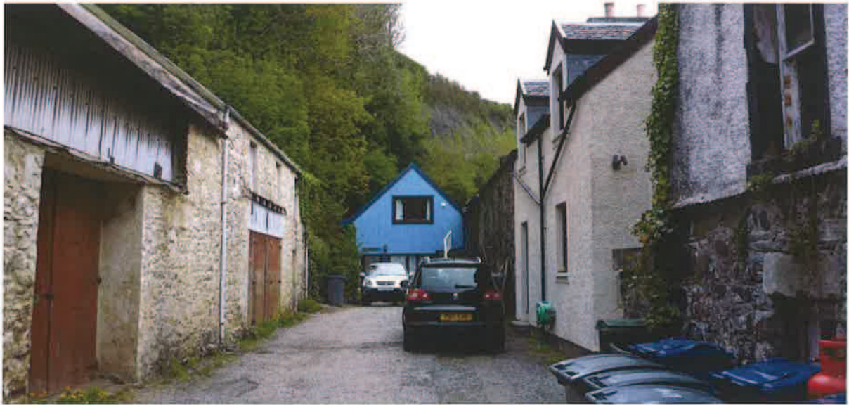
Figure 6 : Just off Main Street, metal/corrugated roof materials and Painted timber house.
