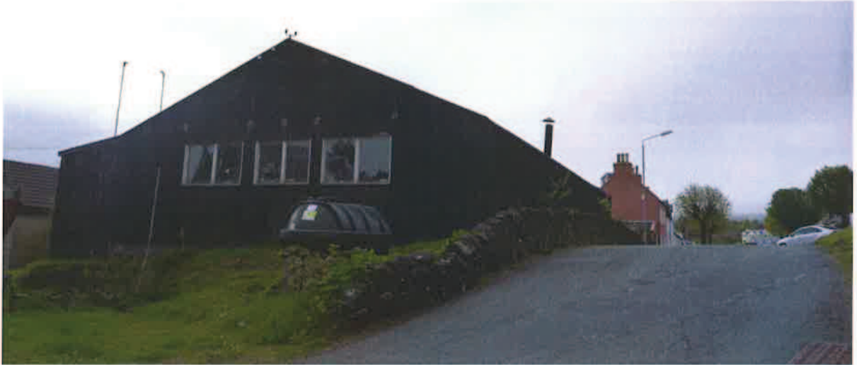
Figure 10 : Corrugated metal roof and wall materials (breadalbane st)
