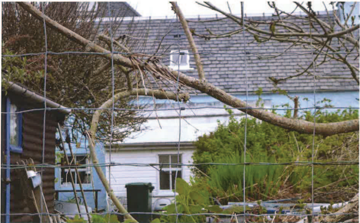
Figure 13 : Timber Clad, Metal Roofed extension (Victoria St)
