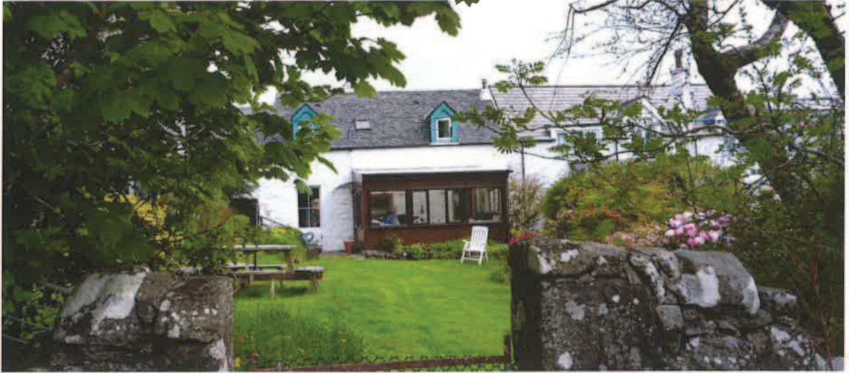
Figure 16 : Timber Clad, Plastic Roof (Albert St)
