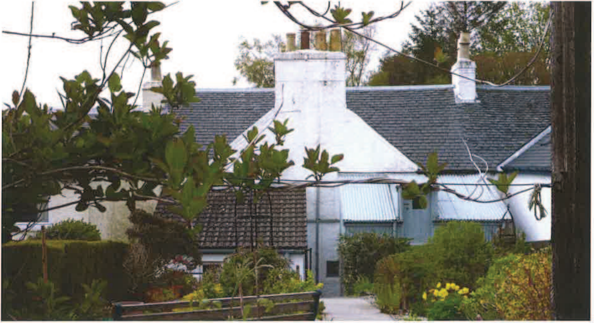
Figure 14 : Corrugated Metal Extension (Albert St)
