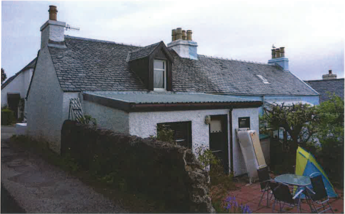
Figure 12 : Profiled metal roof (Victoria St)
