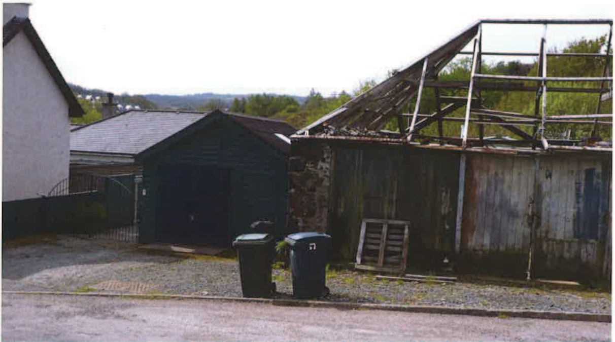
Figure 19 : Timber Garage with corrugated roof (beside, until recently, metal roofed building) on main street scene
