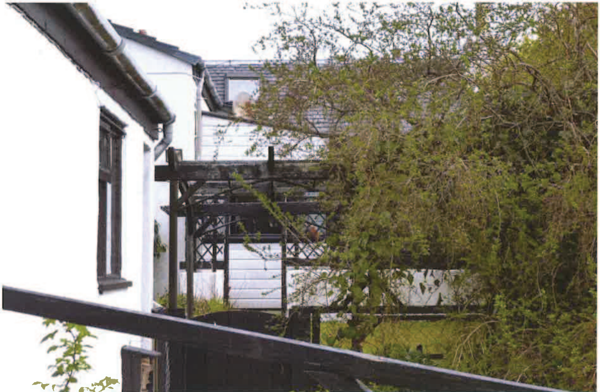
Figure 15 : Timber Clad, Felt Roof Extension (Victoria St)
