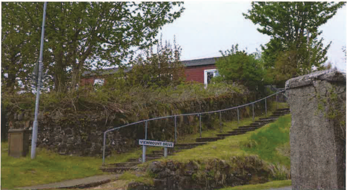
Figure 9 : Corrugated roofing and Timber Cladding on building just off Viewmount Drive
